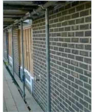
Section of brickwork where joints have been cut and cleaned out.
