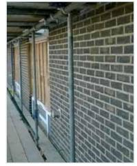
Section of brickwork where joints have been cut and cleaned out.
