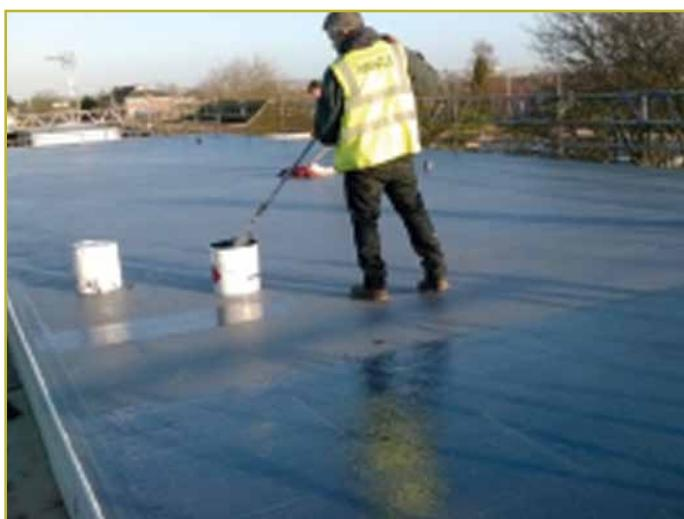
*The roof at 1-9 Mill Lane receiving its final coat of the Proteus system*
