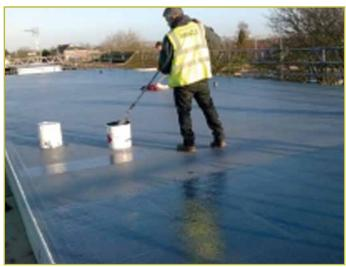
The roof at 1-9 Mill Lane receiving its final coat of the Proteus system
