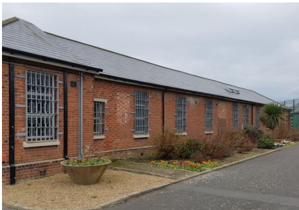
The barrack ranges showing the southern most slightly projecting bay and precise rhythm of elongated openings with rubbed brick lintels and stone cills. Under floor ventilation can be seen within the plinth.
