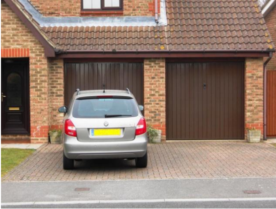
These garages are too narrow for a car and the driveway is too short to allow convenient access for cycle storage.
