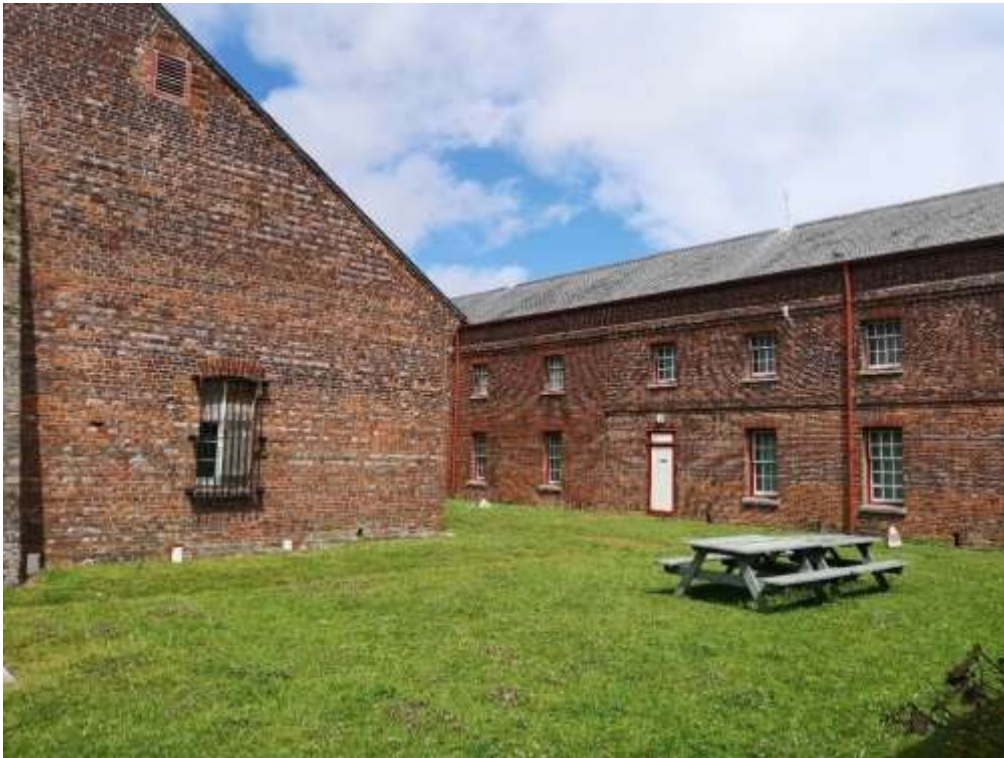
Figure 25 Red brick with burnt headers and natural slate are the prevailing historic building materials
