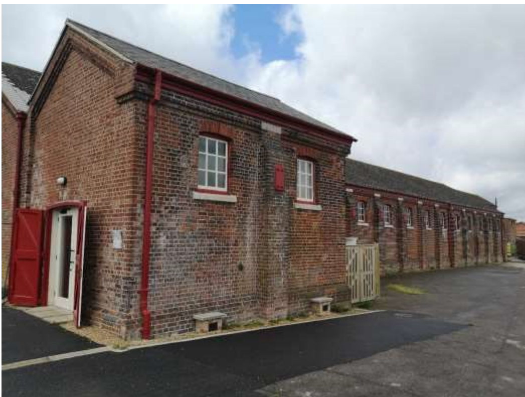
Figure 24 Brick corbelling, buttresses and multi-paned timber-framed windows
