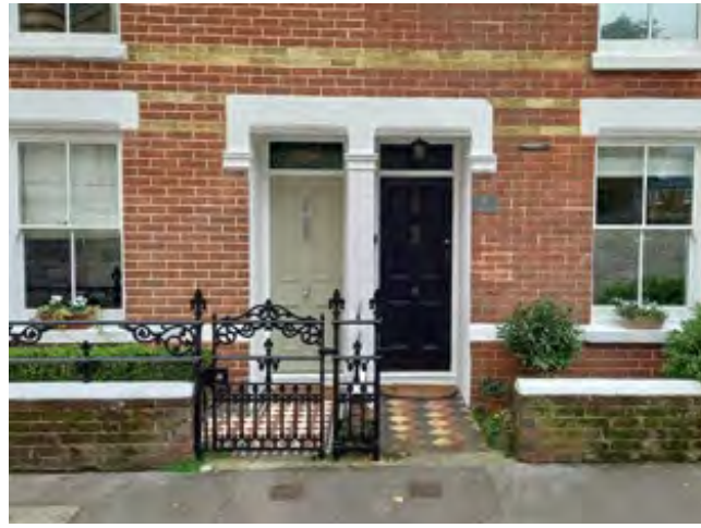
4.9 Polychromatic brickwork and chamfered stone lintels on C19th terraces.
