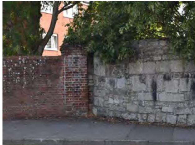
4.19 Combination of stone and brick walls
