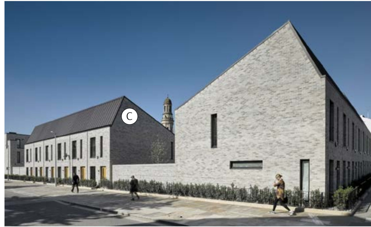
Timekeepers Square, Buttress Architects
