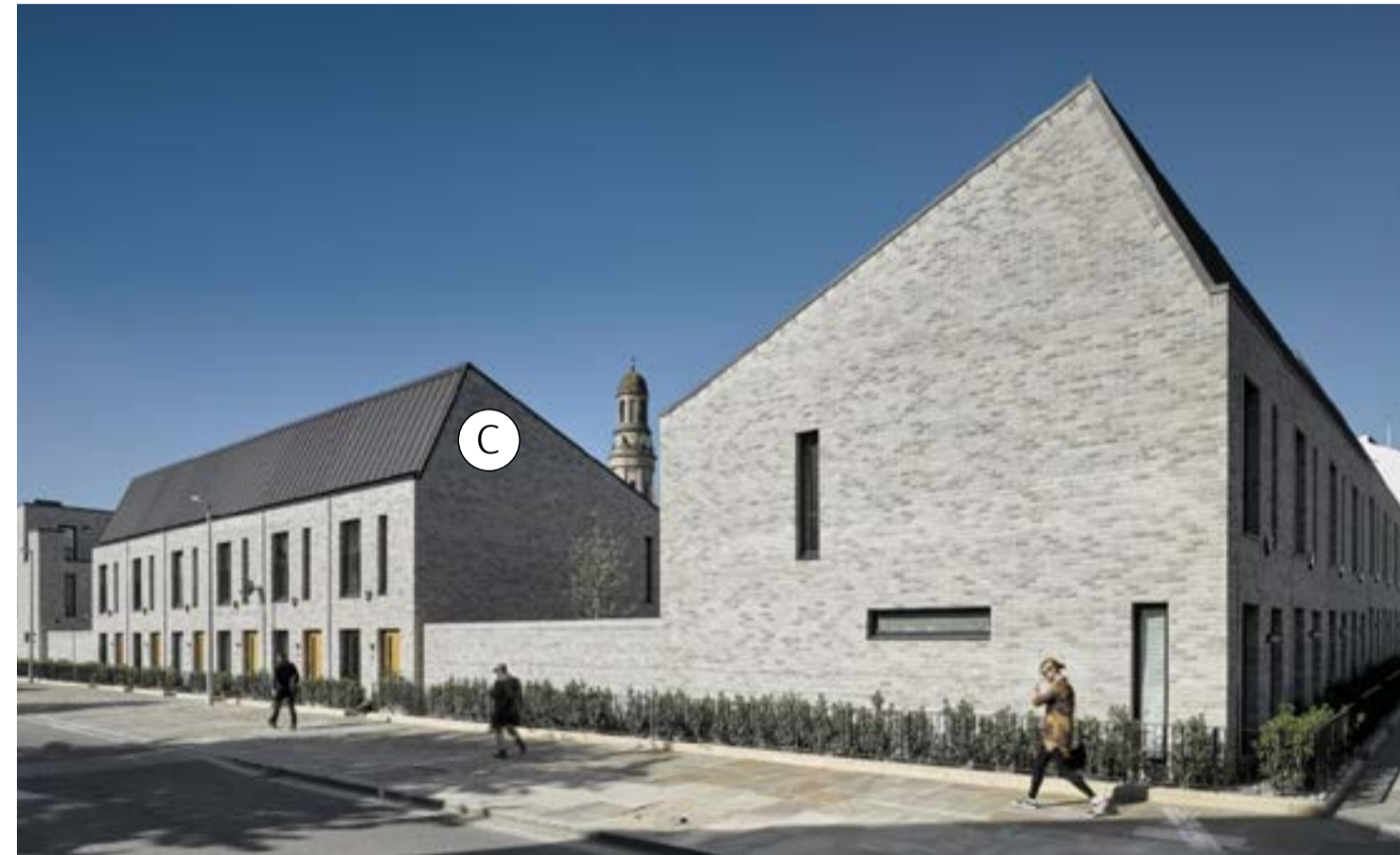
Timekeepers Square, Buttress Architects
