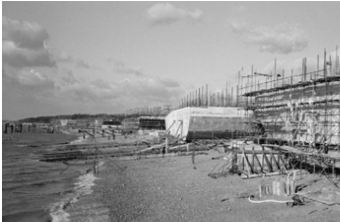
3.43 Phoenix caissons under construction at Stokes Bay (fortgilkicker.co.uk).
