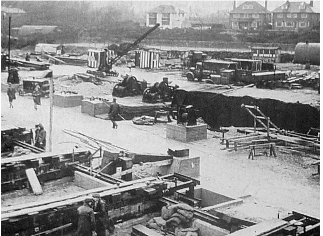
3.44 A slipway under construction at the western Phoenix construction site at Stokes Bay (fortgilkicker.co.uk)
