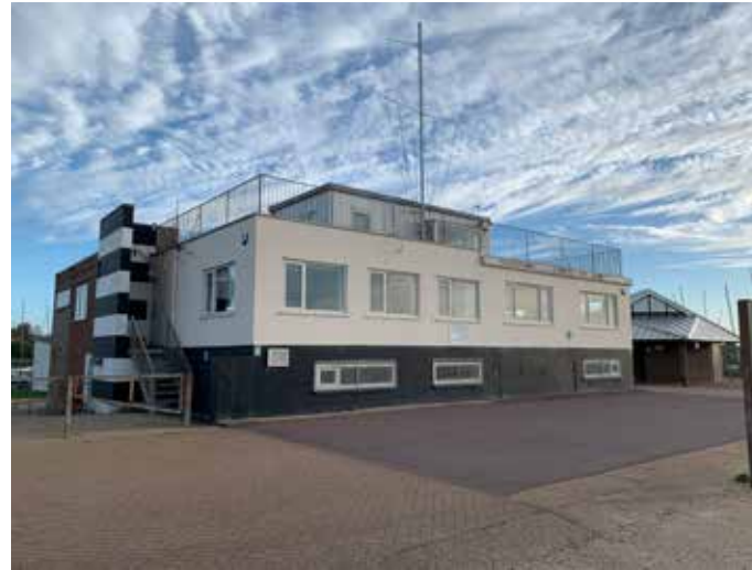
4.4 Former D-Day Control Centre
