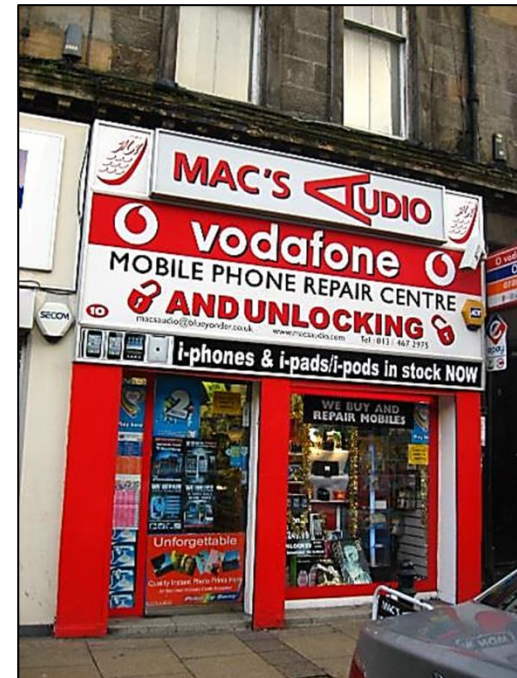
Fig 6: Fascia is disproportionate to building and shopfront design
