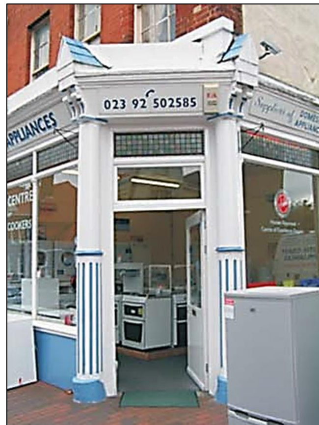
Fig 7: Detail of an historic shopfront on Stoke Road
