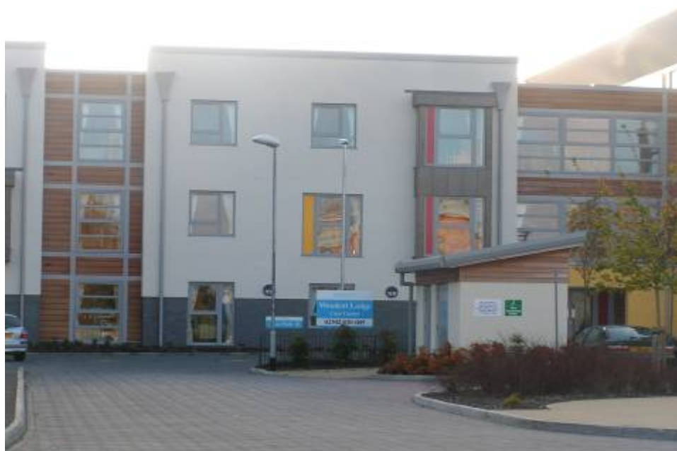
Figure 9.1: Woodcot Lodge Care Centre
