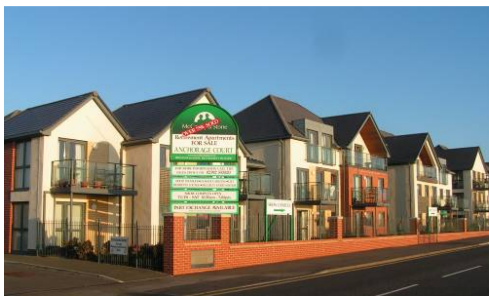
Figure 6.17: Anchorage Court is an example of a scheme that scored highly
