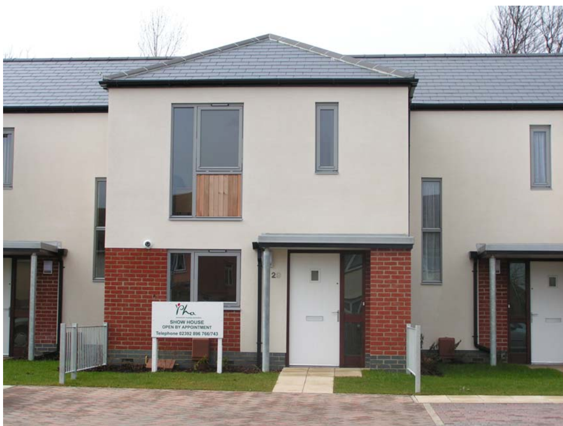
Figure 6.2: New affordable housing at James Road, Gosport
