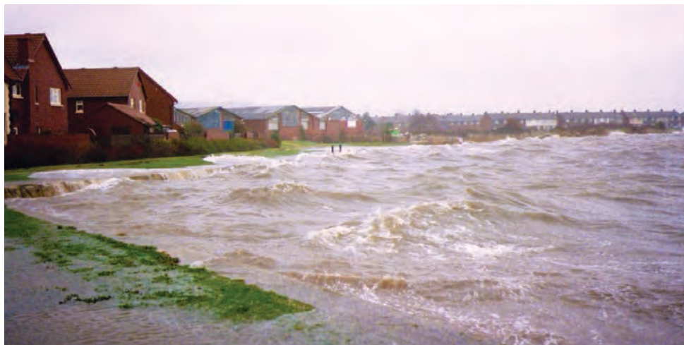
Wave overtopping during a winter storm at Cadour Drive
