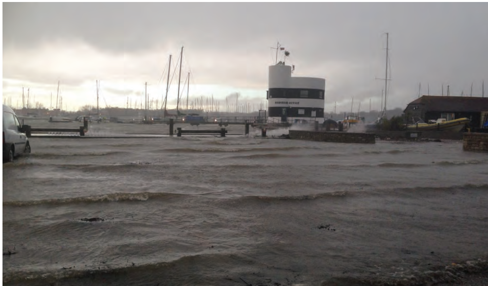
Flooding of the car park at Warsash during the February 2014 storm
