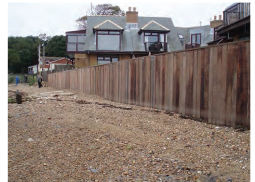
Timber Clad Sheet Pile Wall
