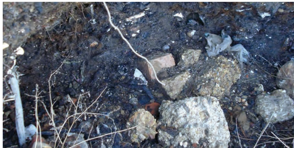
Erosion of potentially contaminated land at Wicor Recreation Ground
