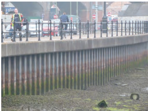
Steel Sheet Piling
