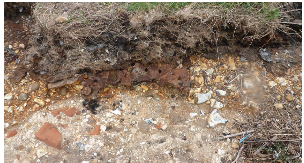
Former landfill eroding along the northern shore of Portsmouth Harbour
