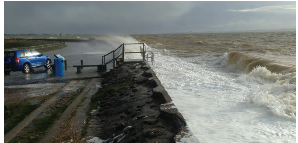
Wave overtopping near Hill Head Harbour during a storm
