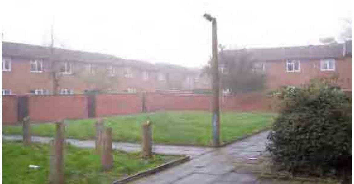
Figure 2.2 A poor-quality space with a layout where pedestrians and vehicles are segregated. It has not been a success and the area is now undergoing regeneration.
