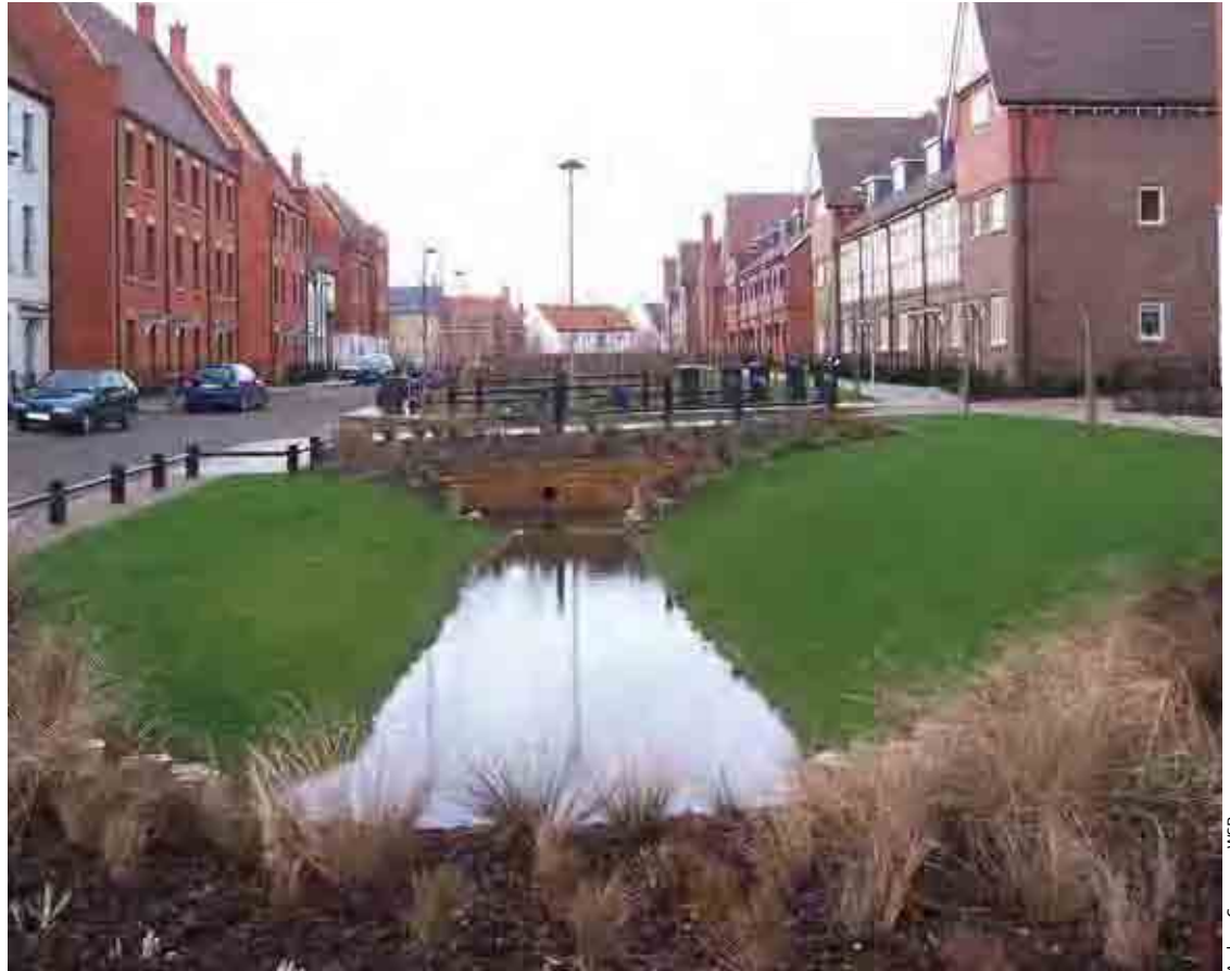
Figure 11.5 Sustainable drainage systems can form an integral and attractive part of the street.
