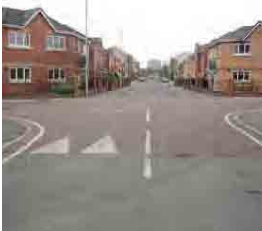
Figure 7.13 Raised tables at junction in Hulme. The table has been raised almost to kerb height.
