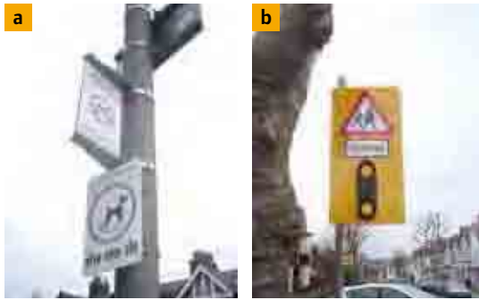
Figure 9.1 (a) Sign clutter in residential areas; (b) the yellow backing board adds clutter and its use with the flashing amber lights is counter-productive. In addition, the sign post should not protrude above the sign.
