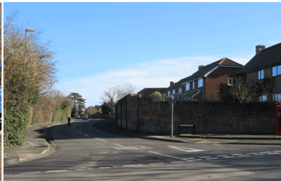
High walls – Clayhall Road
