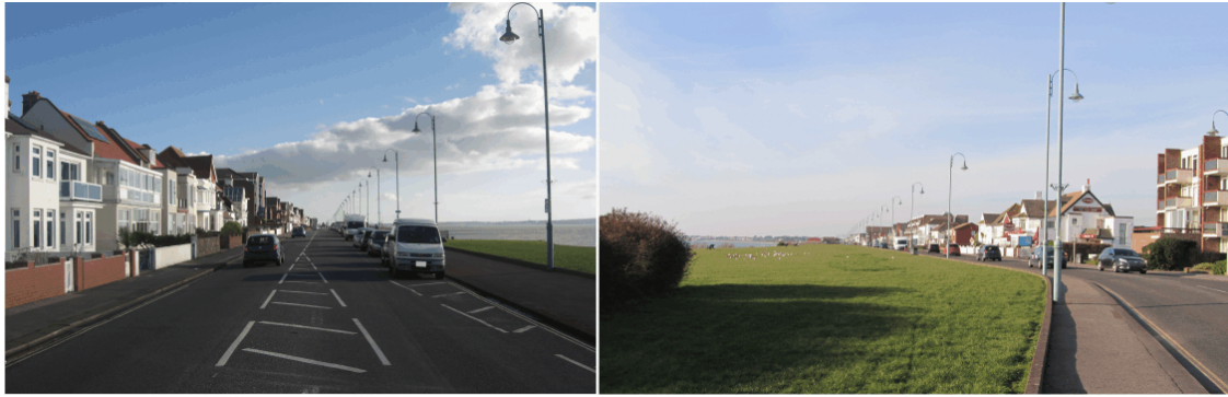
Marine Parade west end frontage - domestic scale Wide verges at the east end
