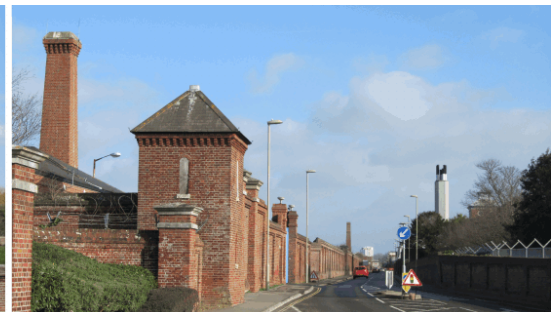
Haslar Road - walls
