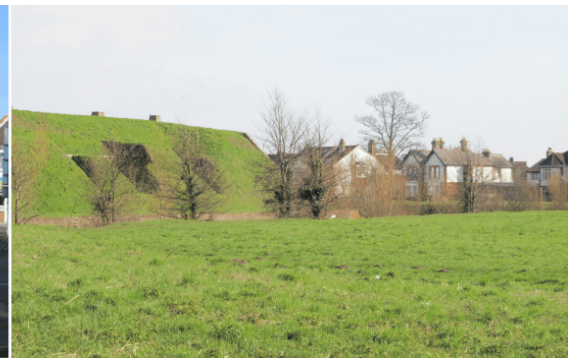
Fort, moat and open space
