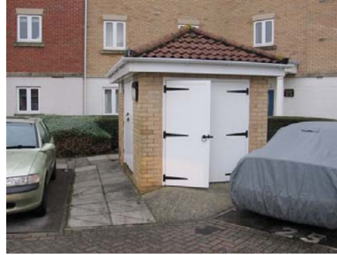
Fig 70 Example of poor storage for communal properties (Car obstructing access, ramp too steep)
