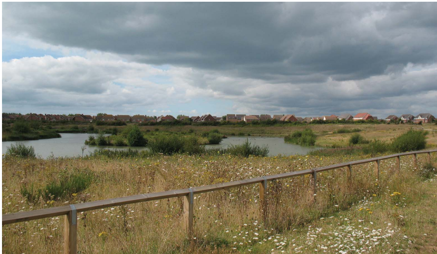
Fig 33: Sustainable Drainage System serving the Cherque Farm development, Lee-on-the-Solent
