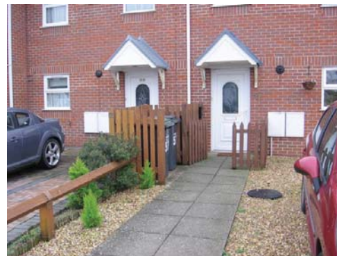
Fig 67 Example of good storage for single dwelling
