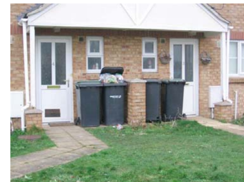
Fig 68 Example of poor storage for single dwelling (no screening)
