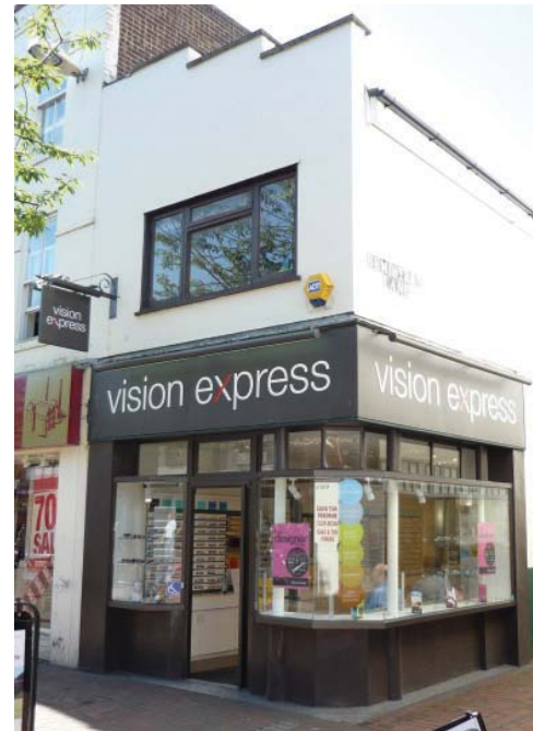
Fig 80: Good example of well proportioned modern shopfront
