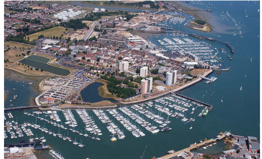
Fig 2: Aerial View of Gosport town centre
